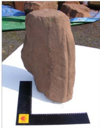
Plate 4, Mouldings on the face of Stone 8, part of a "hood moulding" from the arch of a doorway or window. The moulding has a 45° chamfer on the inner edge and a "V" shaped groove central to the face.
